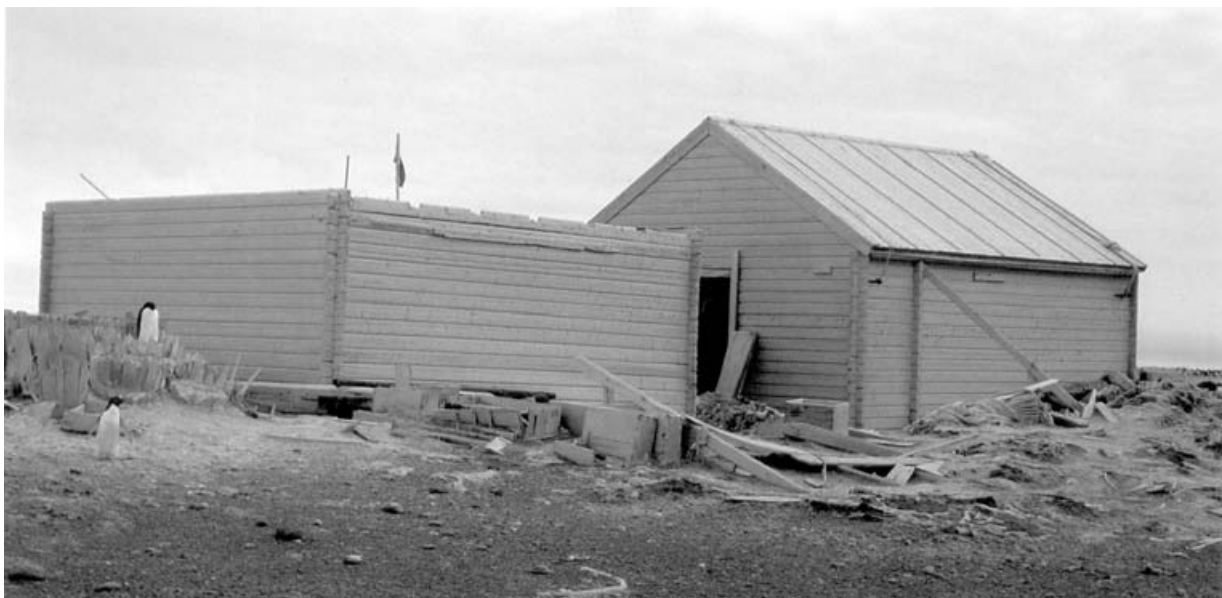
Fig. 3. Borchgrevink's huts, Cape Adare, viewed from the south east. January 1982.
