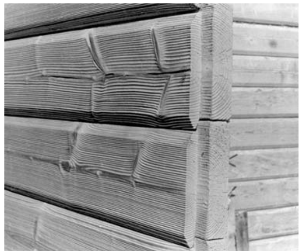
Fig. 5a. Weathered north wall boards, Borchgrevink's 'stores hut'. January 1982.
