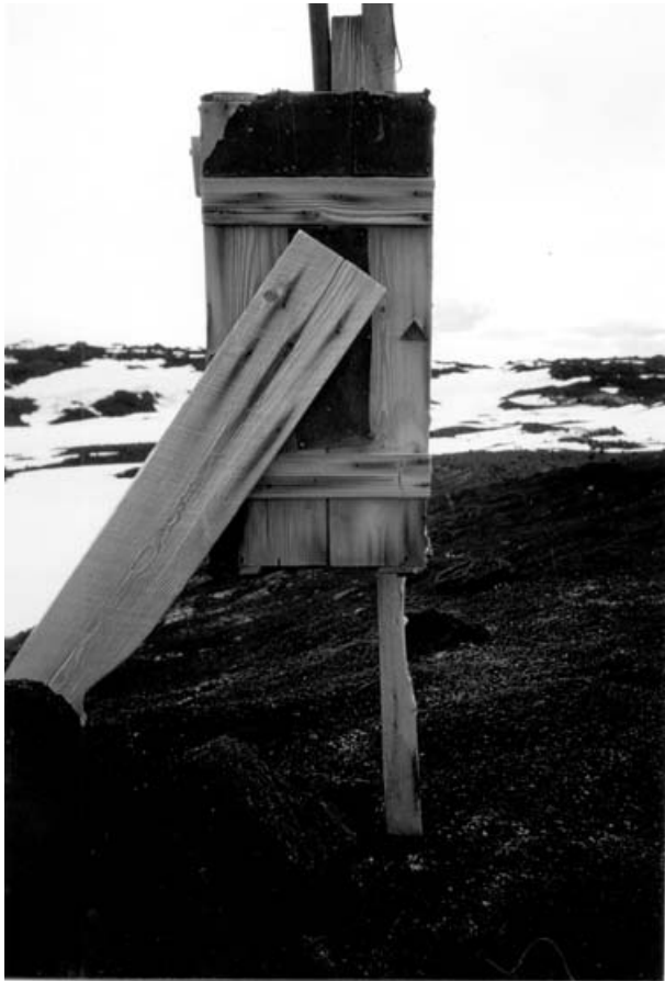
Fig. 14. Weathered instrument housing and support instrument stand, Wind Vane Hill, Cape Evans. January 2004.
